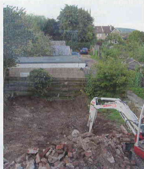
A mini-digger makes light work of excavating the hole for the pond
