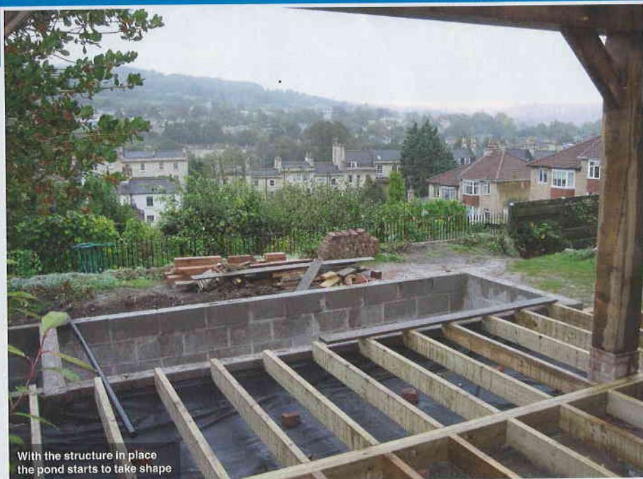
Nick begins the process of installing the liner
